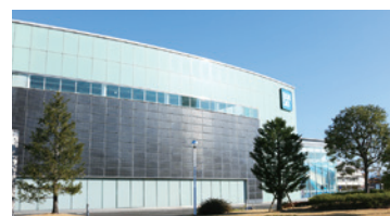
Large solar panels installed on the facility wall
